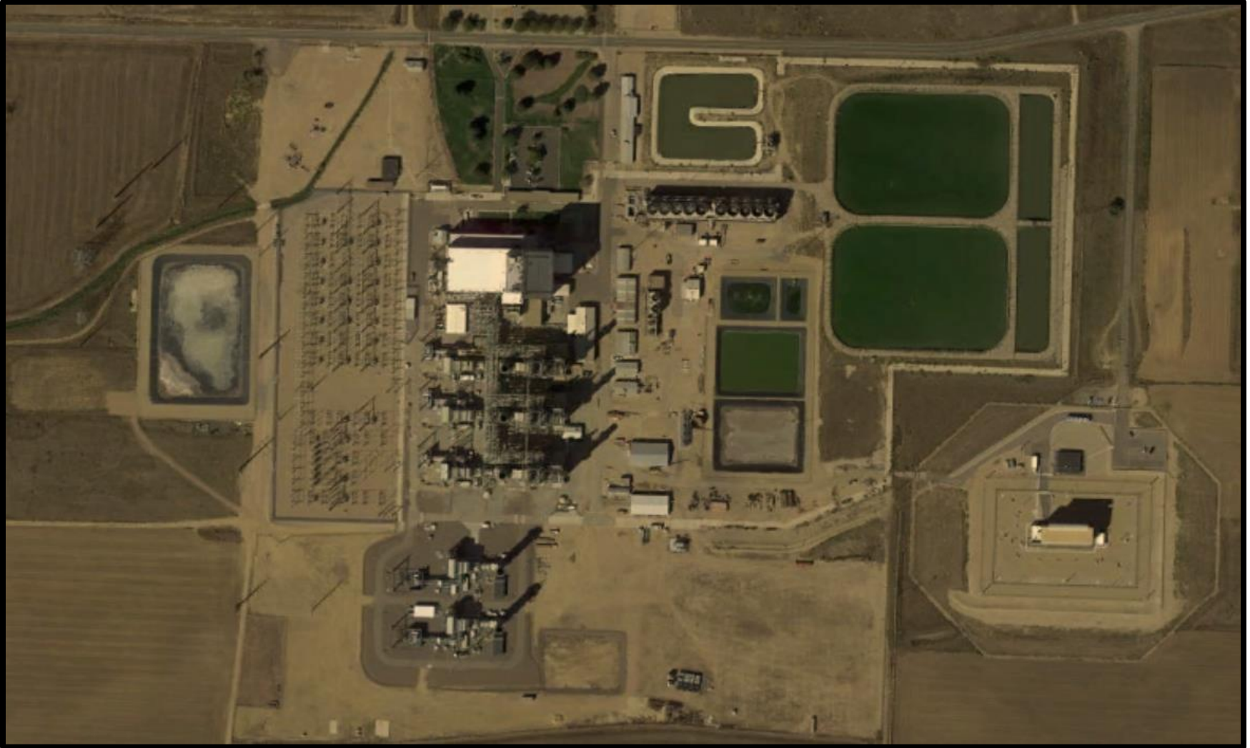
Figure E-3: Fort St Vrain Site Aerial
